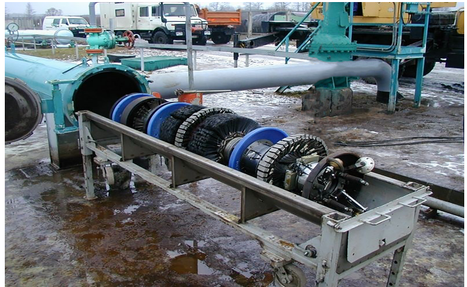
Fig. 1. A pipeline inspection gauge (PIG) is being inserted into a pipe.
