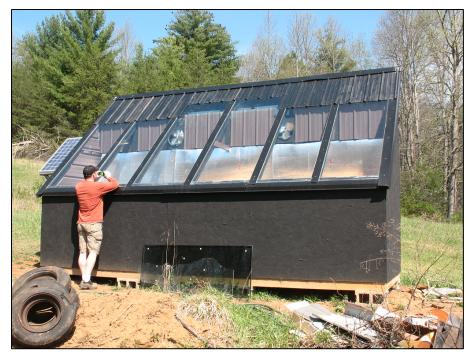
Figure 7. Solar kiln and solar-photovoltaic-driven fans.
