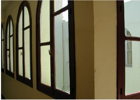
Figure 6: Painting the window's glass constitutes another mean to control daylight and sunlight admission.
