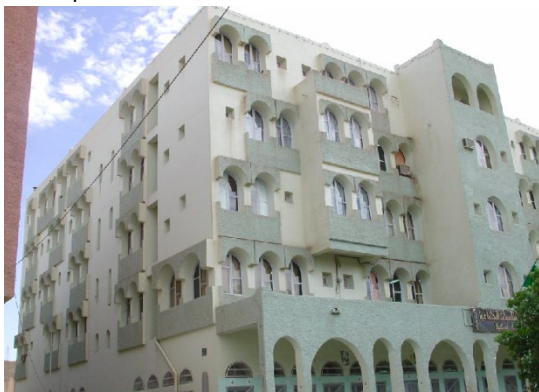
Figure 1: A view of the investigated building: CNAS (Caisse Nationale des Assurances Sociales) showing its various openings.
