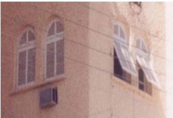
Figure 4: External and internal views on the closed and opened position of the external solar protections (shutters).
