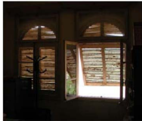
Figure 4: External and internal views on the closed and opened position of the external solar protections (shutters).
