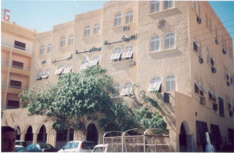
Figure 1: A view of the investigated building: SAA (Société Algérienne des Assurances).
