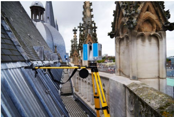
Figure 4. Terrestrial scanning from parapet level.
