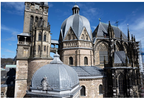
Figure 5. South view of Cathedral roofs.
