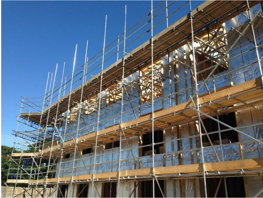
Figure 1. Bloc D in construction
