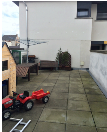
Terrace 6 th Floor
