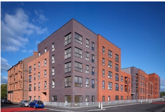
Figure 5.41: Byron Street development designed by Collective Architecture
