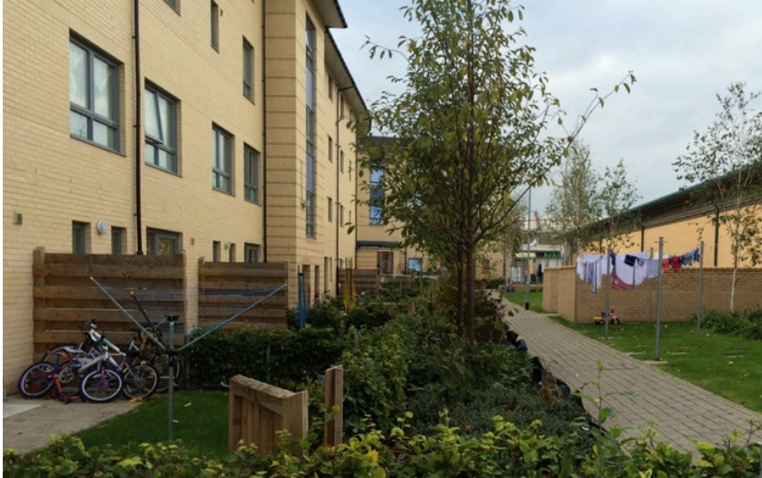
Figure 5.4: Combining back garden and private open spaces – McNeil Development, Glasgow, New Gorbals H.A.
