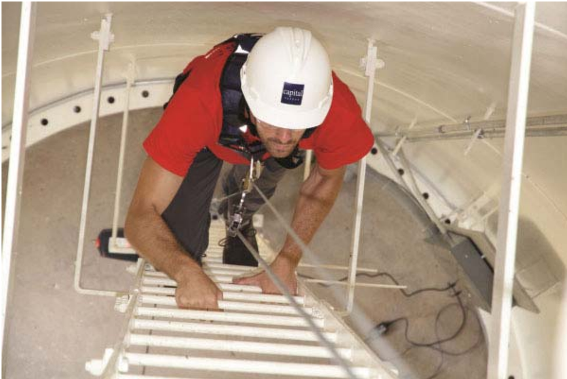
Figure 2. Climb assist system in use (With permission from Capital Safety)
