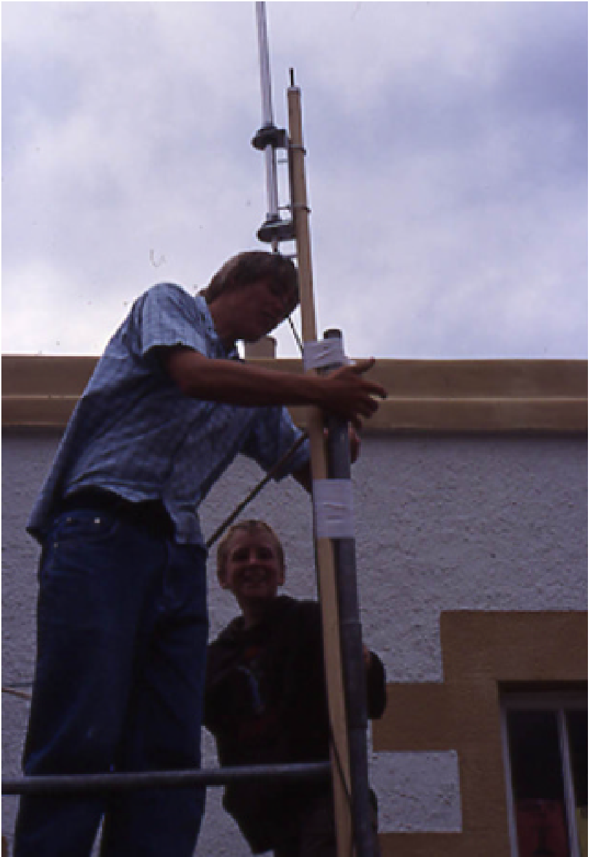
Erecting the antenna prior to the first test transmission.
