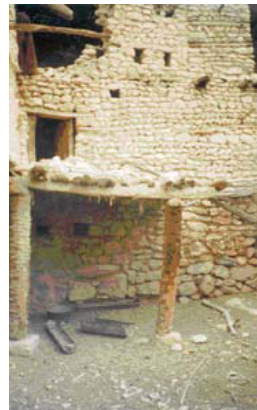
Figure 6: A covered area in the courtyard provides a protected against heat and glare space.
